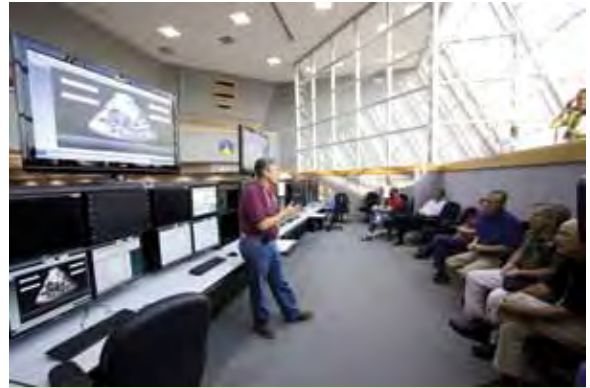
At the newly remodeled Launch Control Center's Young-Crippen Firing Room at NASA's Kennedy Space Center, engineering directorate personnel demonstrate the recently added Space Command and Control System, which will be used for launches of future human space-flight vehicles. In use since the Apollo era, the Firing Room was rewired and received new equipment and furnishings. (Credit: NASA/J. Grossmann)
